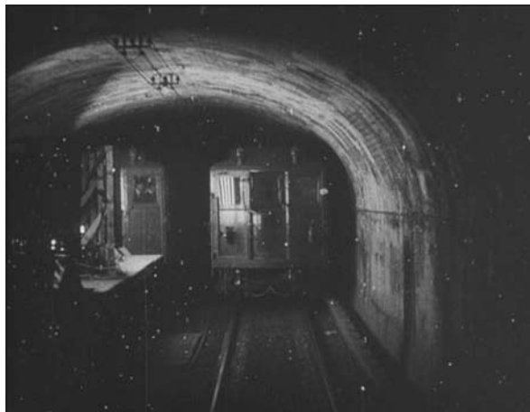
INTERIOR N.Y. SUBWAY, 14TH ST. TO 42ND ST.
